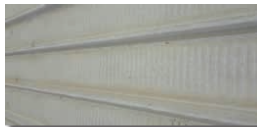
Transverse pan stiffeners
