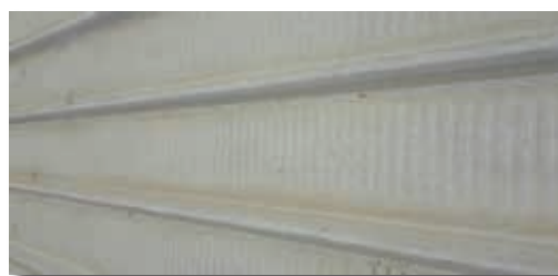
Transverse pan stiffeners
